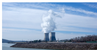
Nuclear Plant—Chattanooga, TN Chemical Cleaning (4) Steam Generators in Reactor Building
