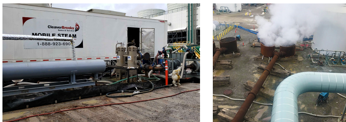
Global EPC's 2x1 Power Generation Facility in Louisiana
